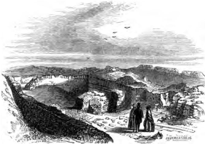
Foundations of a Roman house at Lynne.
